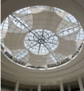
Tensioned sails Lightweight, durable architecture Solar protection under a glass roof
